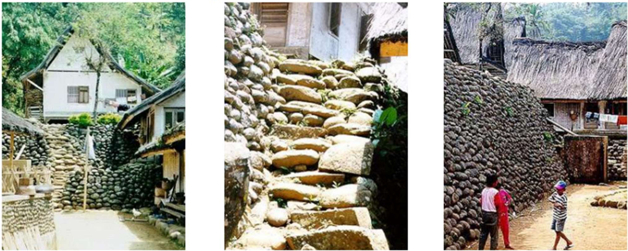
Gambar 07. Dinding batu penahan tanah Sumber: Handayani, S (2009)
