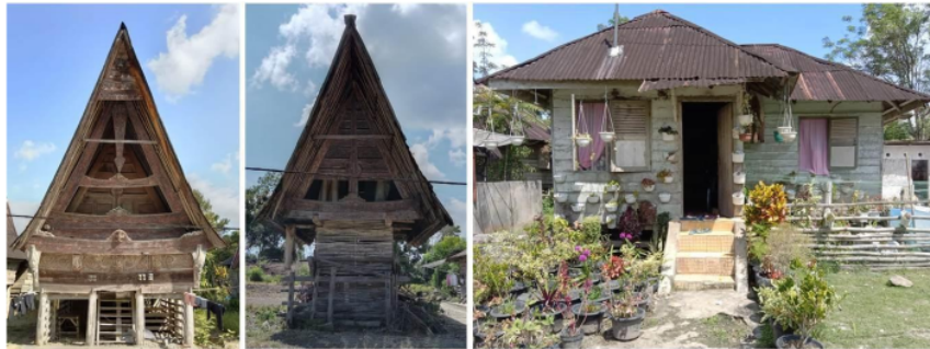
Figure 8. The Building Typology of Sigumpar ( Jabu; Sopo; Ruma Eper ) (Source: Personal Documentation, 2021)
