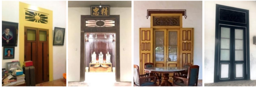
Fig. 6. Doors and Ventilations of Lasem houses
