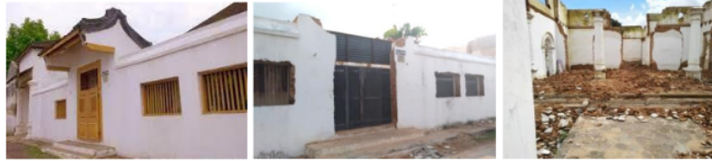
Fig. 11. Karangturi IV/16 Residence Before and after being demolished in 2019
