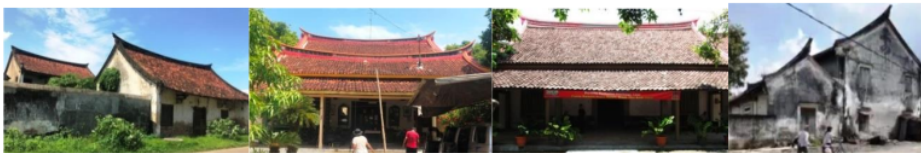
Fig. 3. Early Chinese House Architecture in Soditan Village Source: M. Maria Sudarwani, Edi Purwanto, R. Siti Rukhayah
