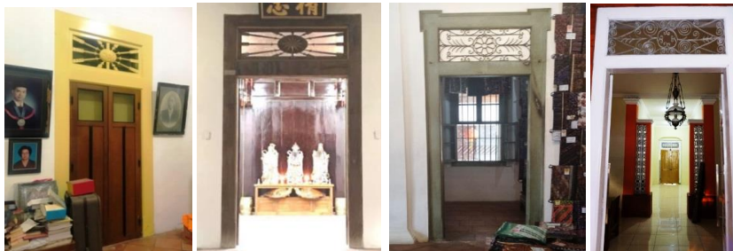
Fig. 5. Various Ventilations of Lasem Door Source: M. Maria Sudarwani, Edi Purwanto, R. Siti Rukhayah
