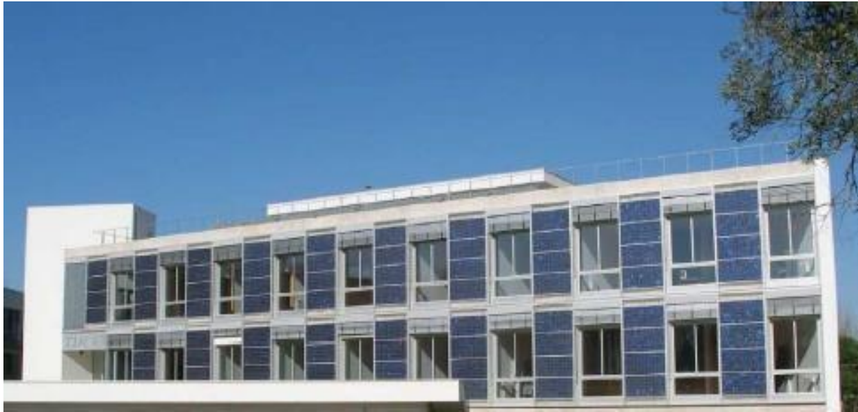
Figure 1. Building Integrated PV (BIPV) (PV- Façade )
