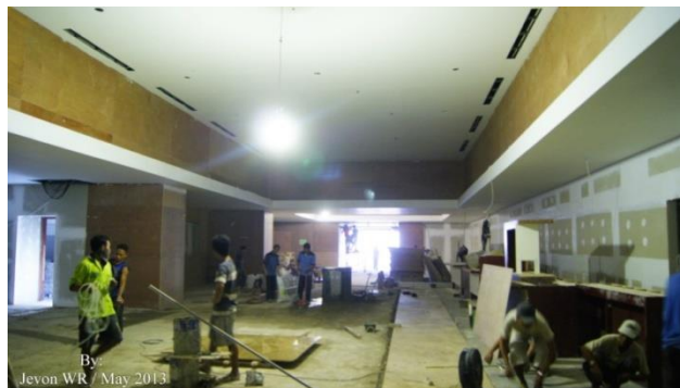
Gambar 11. Pemasangan lantai marmer ( Sumber: http://img59.imageshack.us/img59/4859/dsc07236z.jpg )
