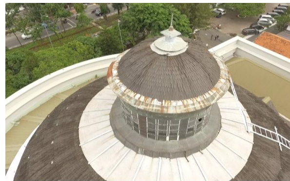
Figure 3. The roof of GPIB Immanuel Church
