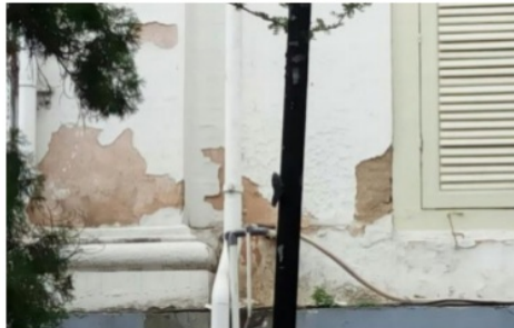
Figure 7. Damage on the outer wall surface
