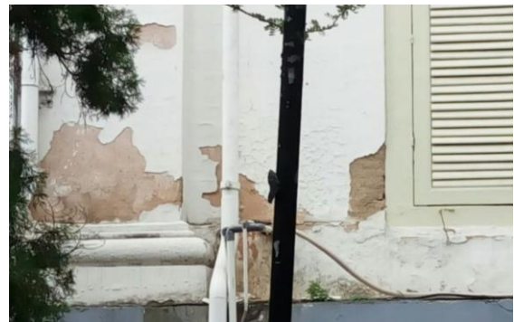
Figure 7. Damage on the outer wall surface
