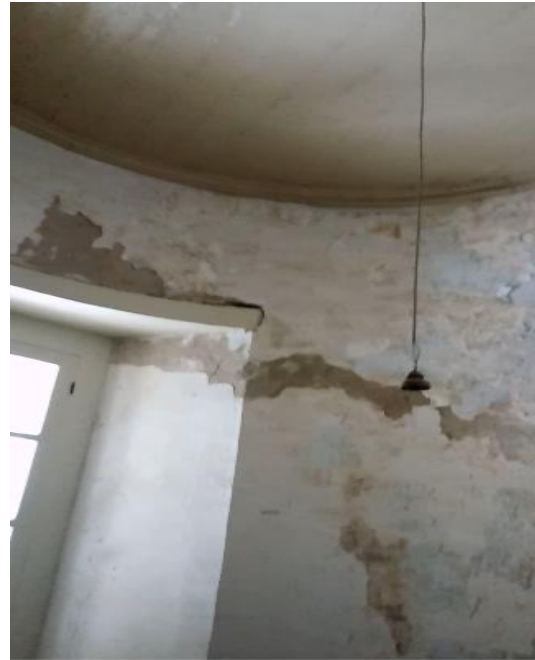
Figure 6. Damage on the inner wall
