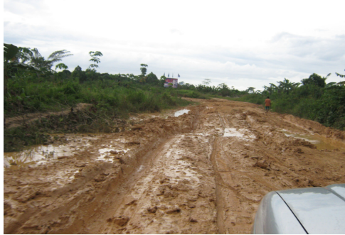
Figure 5. A heavy-muddy surface of roadway
