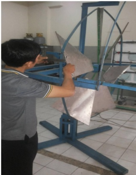
Fig. 2.1. Building and installing wind turbine
