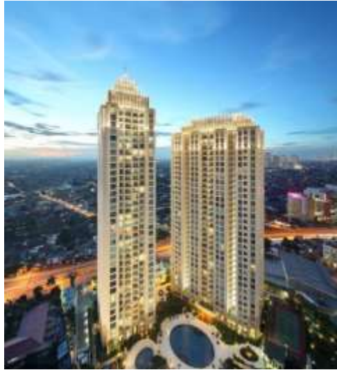
Figure 1. Apartment Pakubuwono Residence
