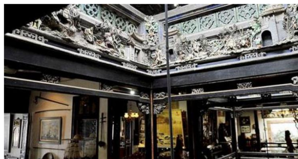
Figure 2. Courtyard and Structural Elements
