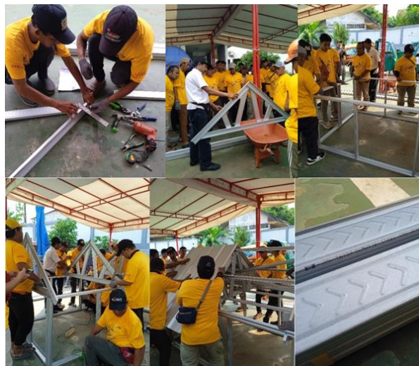
Figure 9. Light Steel Construction Installation Practices
