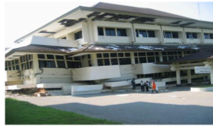
b. Keruntuhan akibat Soft Storey
