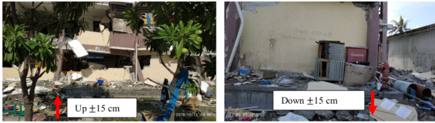
FIGURE 2. Soil deformation pattern due to vertical earthquake (pictures continuous along the length of building)
