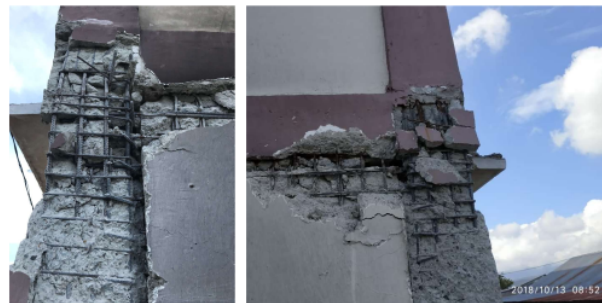
FIGURE 9. Stirrups installed properly in column, beam and joint, concrete crushing because of tension
