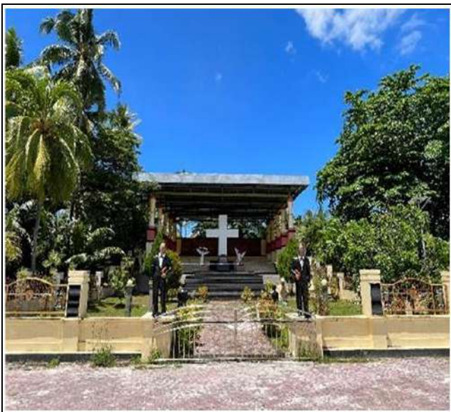
Fig 3 The Condition of the Footpath is not Maintained. Source: Personal Documentation
