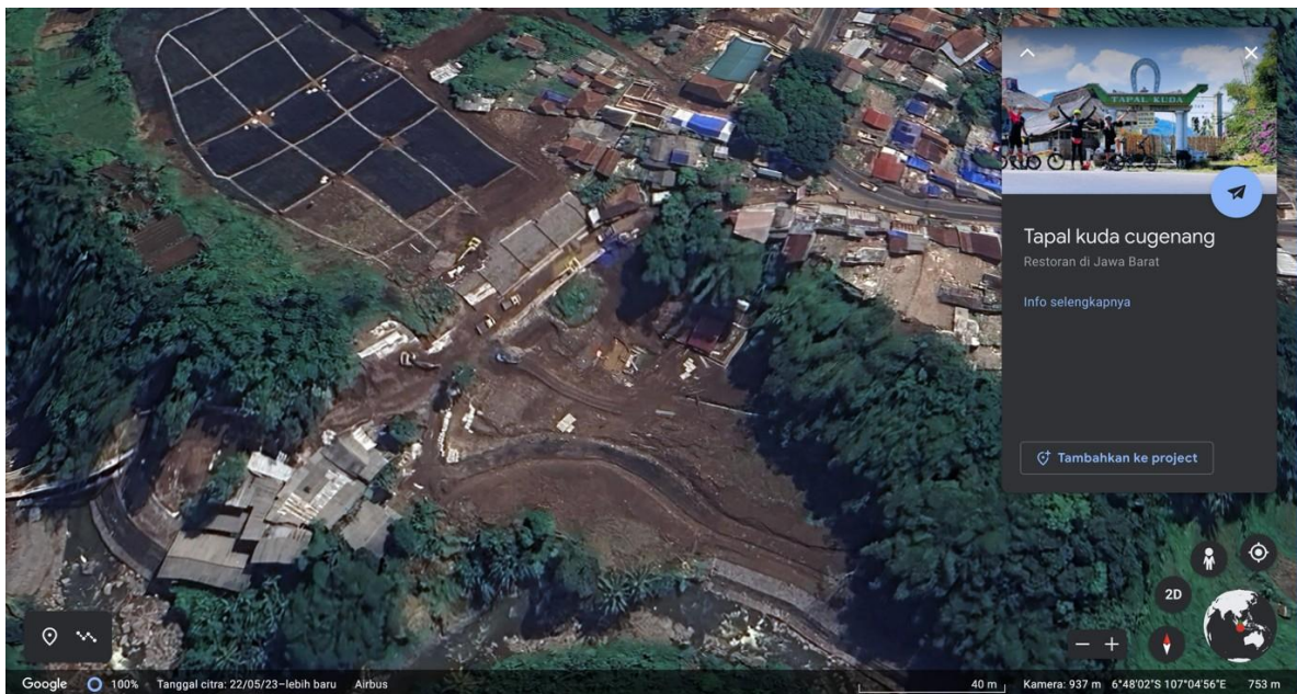
Gambar 1.8. Lokasi Longsor Tapal Kuda, Cugenang, Kabupaten Cianjur (Source: Google Earth)
