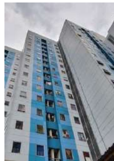
Figure 14. some of window opened when the weather is good.
