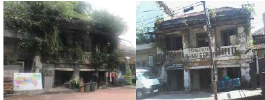
Figure 5. Indies House 2, old and now (Source: Sudarwani & Erwin, 2016; 2023)
