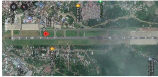
Gambar 1. Lokasi Bandara Sentani, Jayapura (google earth)
