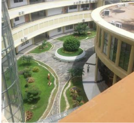
Fig. 15: Inner Yard at Rector and Administrative Office of Padjadjaran University, Jatinangor (Source: www.mldspot.com )
