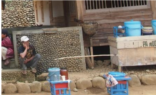
Figure 11. Stone Material used in the House in Kampung Naga
